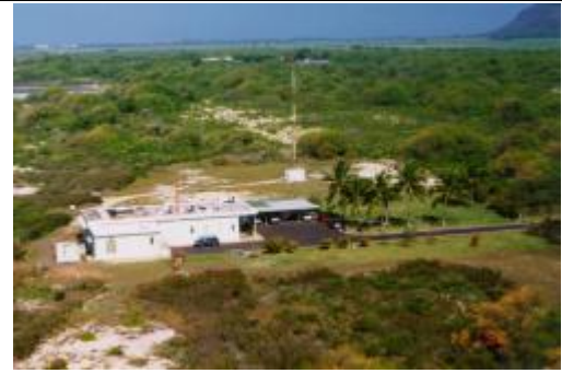
In the Pacific Rim, WWVH in Barking Sands, Kauai is America's second source of time and frequency information. In the foreground is the weather instrument tower, in background, standby 2.5 MHz monopole.
